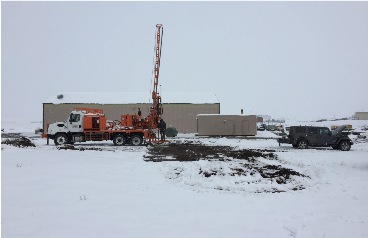
Figure 1: Energy Measurements with Instrumented Subassembly
